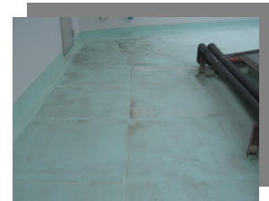
MOSS SCOURING ON THE ROOF
